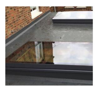
The Frameless Opening Rooflight boasts market leading U-values along with industry leading water tightness using a triple seal gasket system.
